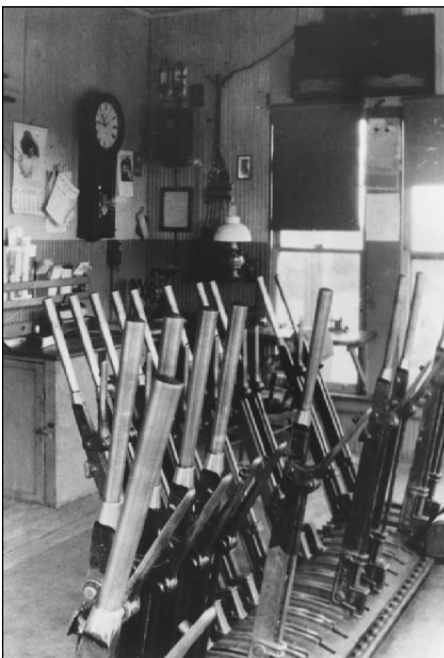
Picture of interior of Woodbine Tower provides a look backwards in time to Sept. 1926. Most of the area inside the tower building was taken up by a series of interlocking, switch and signal control levers. Asher Goldinger photo.
